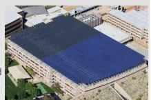
and mechanical components, using state-of-the art software and our well-tuned process for solar power system design. This solution provides the USAA facility with a large fraction of their energy needs while creating the added benefit of providing shade for vehicles parking on the upper level.
